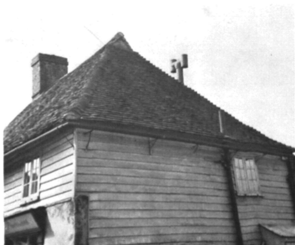
B. Cobham. Wealden-type house. Exterior from S.E. showing gablet.
